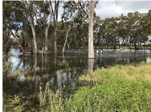
Above: Luckes Weir overtopped and floodwater entering the floodplain (2/11/2022)
